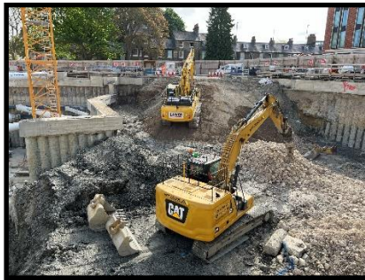
Round Church St bulk excavations & basement slab preparations
