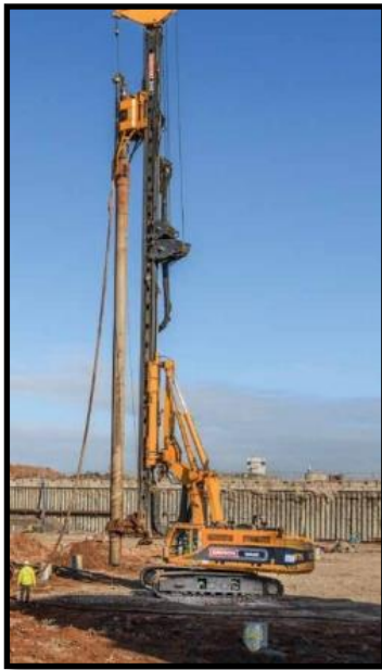
Processing of demolition arisings and preparation of formation levels & piling mat
