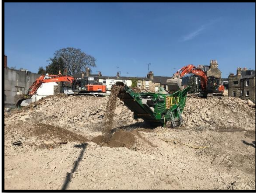
Processing of demolition arisings and preparation of formation levels & piling mat
