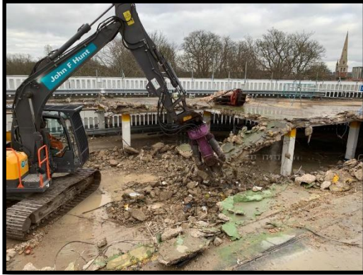
Demolition jaws pulverising & removing slab sections floor bay at a time
