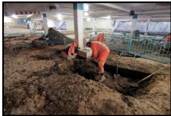
Removed sections of car park slab and ongoing Archaeology in the lower basement area.
